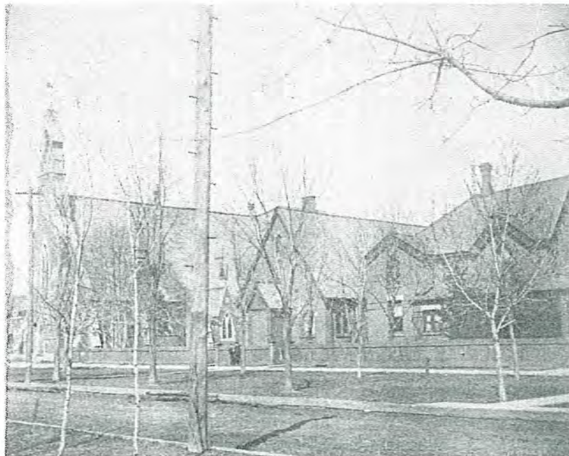
Cedar block curb and roadway in state of disrepair St. Stephen's Church, parish hall relocated and rectory, now both brick veneered, c. 1887 (Metropolitan Toronto Reference Library T30132)
